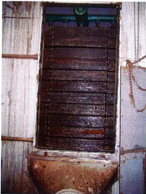
Access Panel Removed
